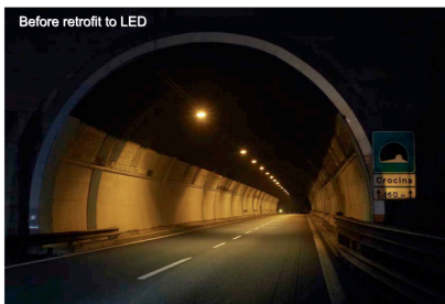
Figure 9: Before LED Retrofit
